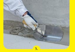
Application with a floor/wall connection: Create a groove with the watertight mortar webertec 933 in the angles between floor and walls.
