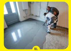
The material is poured from one lane to another one without delay "wet-in-wet".
