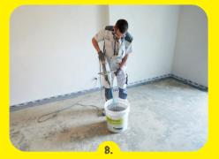
Mixing of the self-levelling and watertight compound. Mix with water until a well flowing and completely lump-free mortar is obtained.
