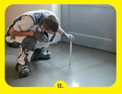
Check of layer thickness: webertec 932 is applied in one layer in thicknesses of 5–30 mm, depending on requirements and substrate. On brick floors the minimum layer thickness is 15 mm.
