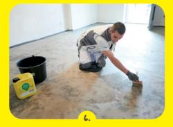
**Priming of mineral substrates:** Apply the bonding primer **weber.prim 932 P**. It is mixed 1: 3 parts by volume with water and brushed intensively thoroughly full-surface into the substrate.
