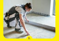
Flatness check and subsequent calculation of layer thickness and material requirements.
