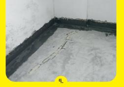
After priming, apply a waterproofing layer of **weber.tec Superflex D 24** on the pre-said connection area and also on the floor along the walls in a width of approx. 20 cm.
