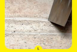
Substrate preparation: Check substrate for sufficient load-bearing capacity. Remove adhesion-impairing components.
