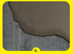
Protection against moisture and radon gas: In this case the whole floor surface is waterproofed with **webertec Superflex D 24** in a dry layer of 4 mm thickness prior to application of **webertec 932**. After drying, **webertec 932** is applied in one layer of at least 10 mm thickness without primer.
