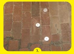
**Priming of brick substrates:** Use **webertec 941** as blocking primer. It is used fullsurface in 2 coats undiluted and intensively brushed onto the substrate.
