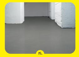
The finished surface can be walked on after approx. 3–5 hours; after final hardening it is open to full load after 7 days and fully abrasion-resistant, e.g. directly usable as wear layer and resistant to chair castors.
