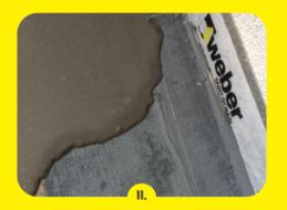
weber.tec 932 is applied without primer on the overlapping area with weber.tec Superflex D 24 on the 20 cm wide stripe along the walls.
