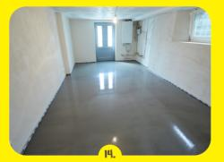
Finished, level and even surface after completion of the levelling and waterproofing works.
