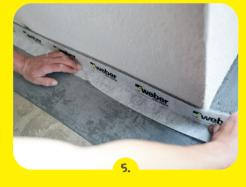
Application without a floor/wall connection: After the waterproofing layer has dried through install the self-bonding acoustic insulation strip weberfloor 4960 along the walls.
