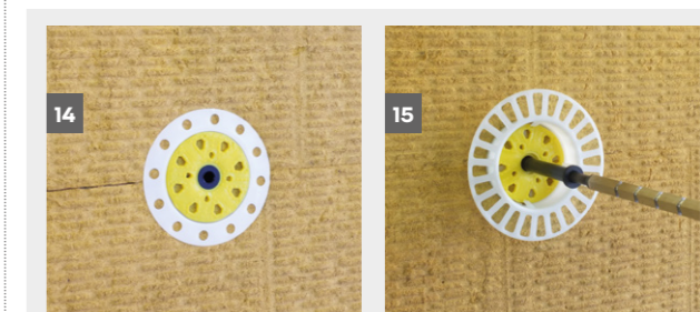
Pic. 14: weber.therm SRD-5 with 90 mm washer (flush with insulation)
