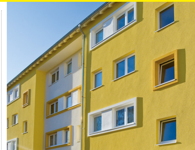
Etics with mineral wool lamella or mineral wool insulation boards and selected mineral overlay renders
