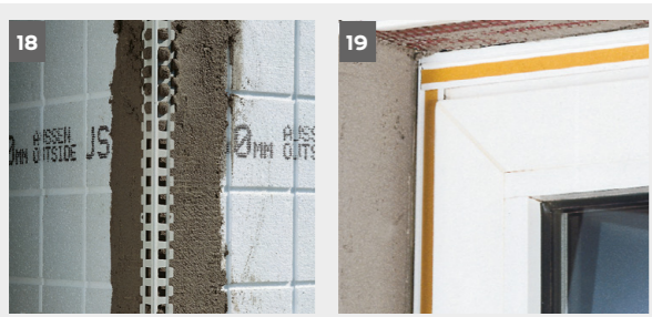
Etics with EPS insulation boards with thick-layer mineral render set-up
