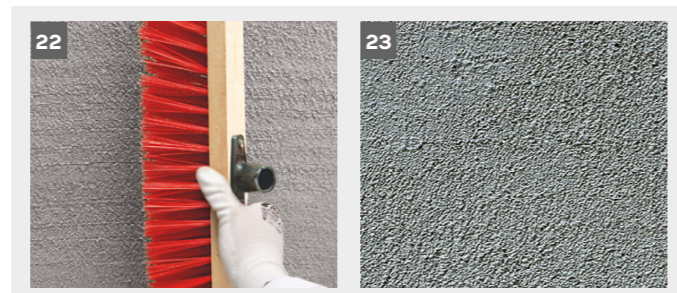
Etics with EPS insulation boards with thick-layer mineral render set-up
