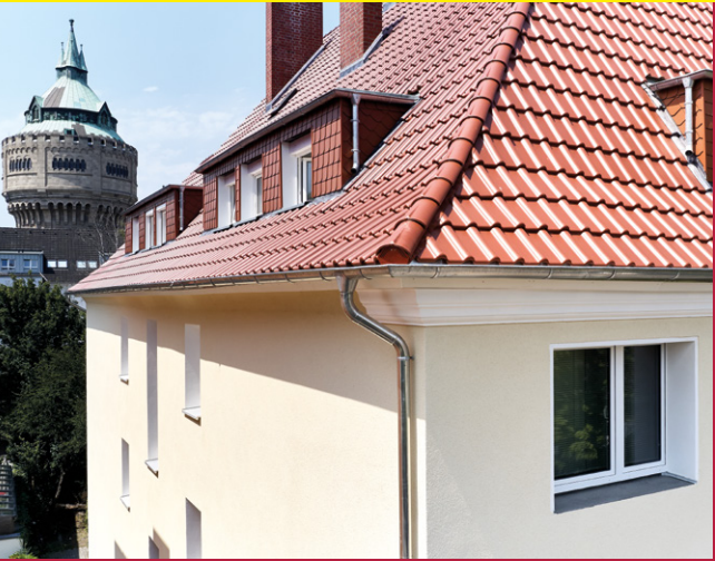
Dismantable ultra thick-layer Etics with mineral wool insulation boards
