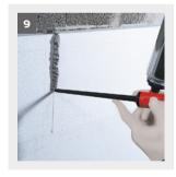
Do not put mortar into the joints between the boards so as to avoid thermal bridges. Even in case of correct processing, it is not always possible to avoid joints in such areas. Fill the joints with the same insulation material and the thin joints (max.1cm) with the PU foam weber.therm 346 (picture 9).
