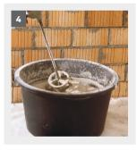
The bonding and reinforcing mortar weber.therm 303 is con-venient for gluing insulation boards. In case of poorly ab sor-bent substrates (for ex. dense concrete or brickwork) use the bonding mortar weber. therm 370. Mix the bag content of the mortar with the specified water quantity, using an electric drill and an appropriate stirrer until the right consistency is obtained (picture 4).
