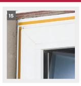
Install a transition between window frame and render with an appropriate frame-seal bead with glass fiber mesh flag, such as weber.therm Gewebeanputzleite (picture 18).
