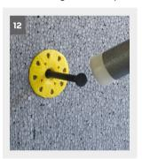
on the substrate install the drive-in dowels weber.therm Schlagdübel (at least 4 pieces per m²). If the stability cannot be obtained in case of non-load-bearing substrates, use the approved screw dowels weber.therm Schraubdübel (picture 12). Always plan 4 dowels/m² in case of timber substrates.
