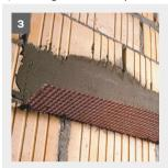
reinforcement weber.therm 312 on the wall with the bonding and reinforcing mortar weber.therm 303, on which the insulation boards will be later bonded (picture 3).
