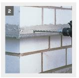
Two possibilities exist: a) Skirting aluminium rail with U-shaped profile: it must match the panel thickness and be fixed with the profile dowels weber.therm 342 (3 pieces per meter) (picture 2). In addition, the skirting rail can be fixed on its whole length with the profile bonding and installation mortar weber.mix 125; this is particularly necessary on uneven
