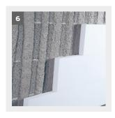
Apply so much mortar that a contact surface with the substrate of at least 50% is obtained after pressing the boards onto the fresh bonding mortar. In case of sufficiently even substrates and in case of insulation boards weber.therm EPS Facade speedy the mortar can be mechanically sprayed in 5 cm-width and 1.5 - 2 cm-thickness beads on the walls (picture. 6).
