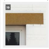
With effect from 2016 in Germany, the fire safety requirements were extended to include the so-called "socket fire scenario". According to these regulations all Etics based on EPS, whatever the insulation thickness is, supplementary measures must be taken to protect the facade from the external side (e.g burning waste container).
