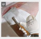
Afterwards lay the woven mesh **weber.therm 311** (fine) in vertical or horizontal wrinkle-free strips across the whole surface. The strips must overlap by at least 10 cm (picture 17). Gently press the mesh with a flat trowel. Afterwards the mesh must lie in the upper half of the reinforcing mortar layer.
