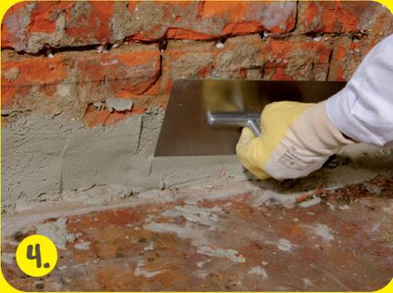
4. Apply **webertec 933** first as bondcoat by brush on the floor/wall connection and afterwards close the created recess with the mortar by trowel.
