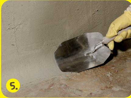
5. Subsequently round out the fillet "wet-on-wet" with **webertec 933**.
