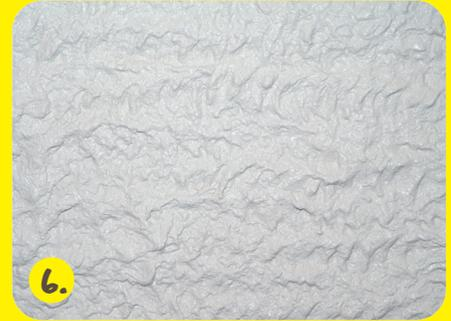
6. Apply a contact layer of the damp-proof restoration render **weber.san 958** over the entire surface of the dull-moist substrate and comb horizontally, preferably whilst still fresh.
