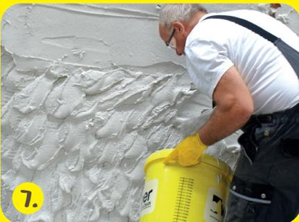
7. Apply the damp-proof render "wet-on-wet" in one layer in thickness up to max. 40 mm.
