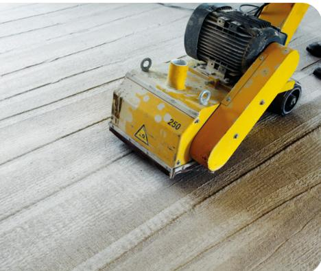
If the substrate is not carefully prepared, even the best flooring system is of no use - the coating cannot form a bond with the substrate and comes off again even under low loads.
