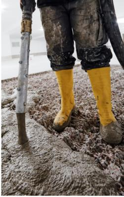
The innovative concrete replacement mortar can be applied up to 48 hours after application of the primer. When applying a bondcoat, this time window is only 20 - 30 minutes.
