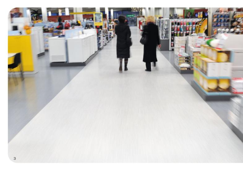
The desired grade of skid resistance can be achieved with the help of scattering mineral fillers (silica sands) that are incorporated into the fresh coating.
